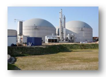
the oxygen is removed. This produces methane when the organic matter breaks down. The methane is then burned, which drives the turbines and creates electricity.
